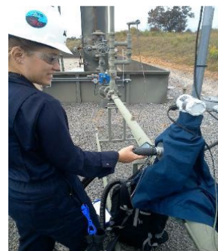
Figure 3: High flow instrument in use. Blue fabric encloses the leak source.
