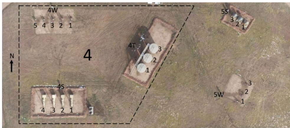
Figure 43: Pad 4 at METEC with equipment groups marked.
