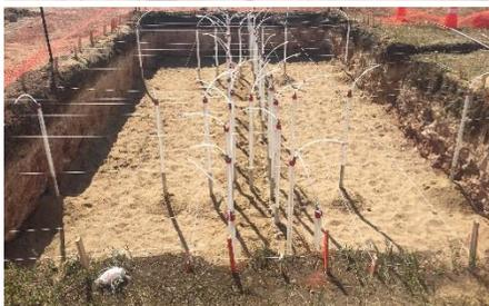
Colorado School of Mines' Dr. Kate Smits, her graduate student Melissa Mitten and a cadre of CSM students worked long and hard hours at METEC with Dr. Clay Bell and Mike McGuire to get the pipeline test bed trenched, piped and instrumented with emission points and sensors. The test bed will provide realistic emission profiles for testing sensor solutions designed for underground leak detection. The test bed emissions will be controlled in
