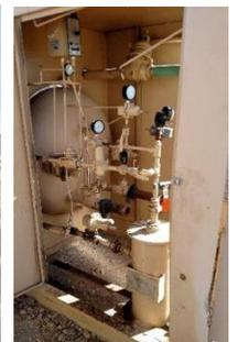
**Functional Components Are in Place.** The compressor system for the field site has been established. A Norwalk compressor installed at the Powerhouse Energy Institute and capable of 60 SCFM at 3600 psi will provide CNG for the test site. The compressor system will incorporate 60 GGE of storage to allow rapid fill or time fill of the CNG transport vehicle.
